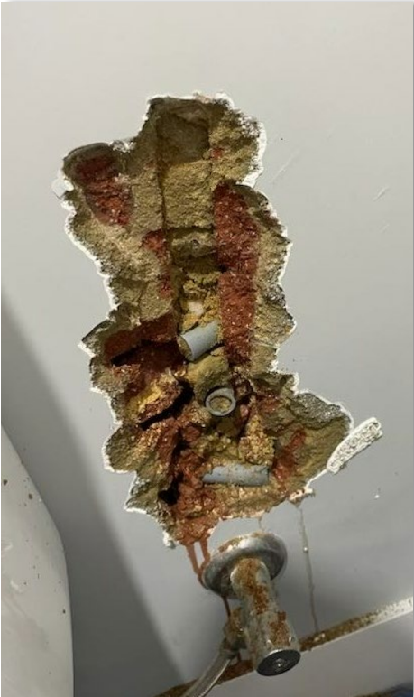
Pinch/pressure point caused by pegging creating localised high stresses
