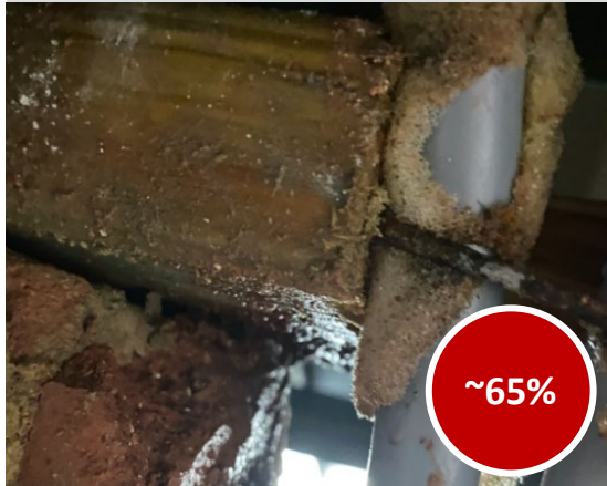
Pipe bend across metal nail and kinked, resulting in a stress point
