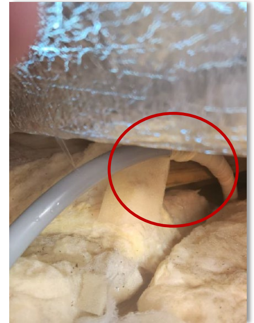
The bend of these pipes are likely to be outside of Iplex Pro-fit instructions (too tight), placing stress on the pipes
