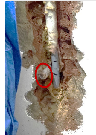
Inadequate movement and damage to pipe caused by pegging left in chase
