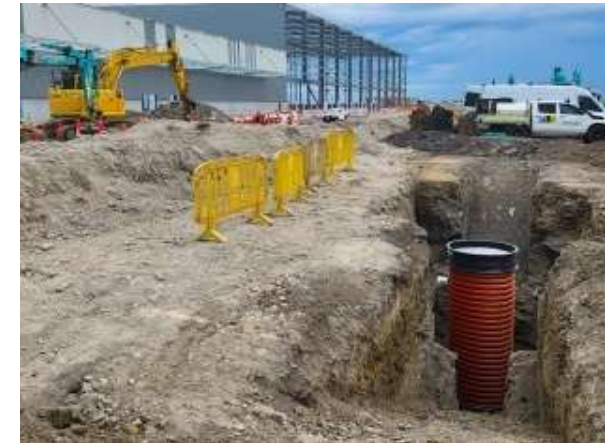
Western Sydney International Airport – Iplex AU
