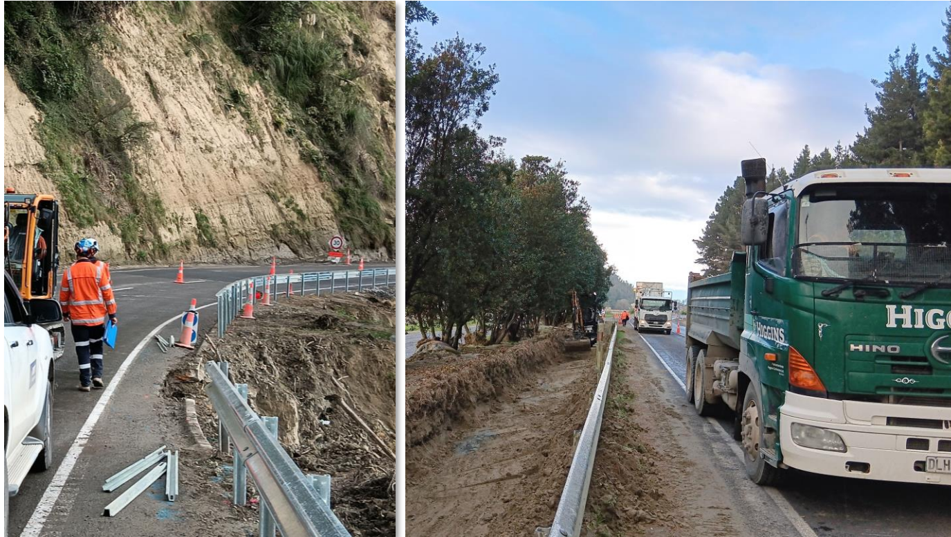
Remediation of significant damage to critical roads
