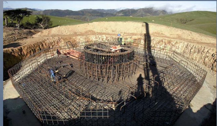
48 tonnes of steel in each 15m base of the 112m high Makara turbines
