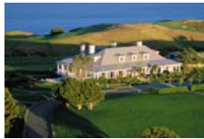
PCC Coil on Kauri Cliffs Roof
