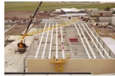
Long Span Commercial Roof and Purlins
