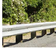
Coating on Armco Railing
