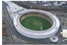
Westpac Stadium Cladding and Roof
