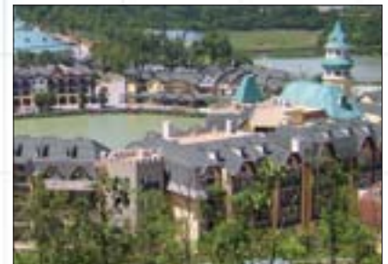
A major complex emerges with the help of AHI Roofing in Shenzhen city, near Hong Kong.
