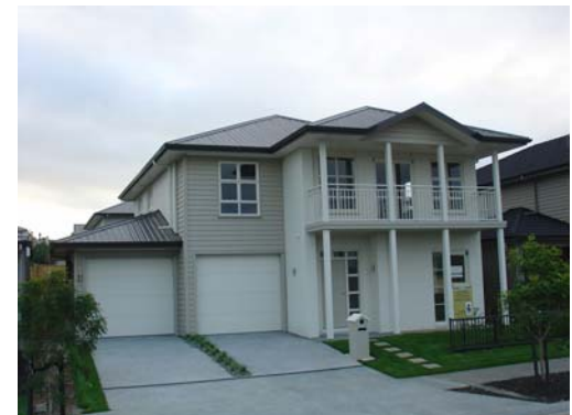
New house built by Fletcher Residential in Auckland, 2007
