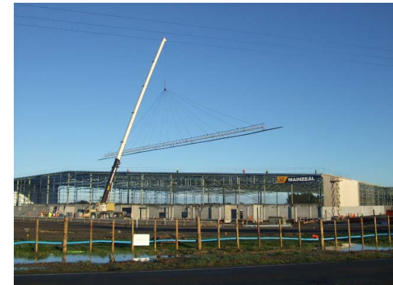
88 metre long Dimond sheets, Palmerston North 2008.
