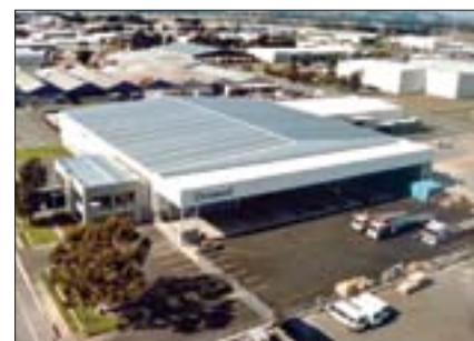
Dimond's new facility in Christchurch, completed during the year.
